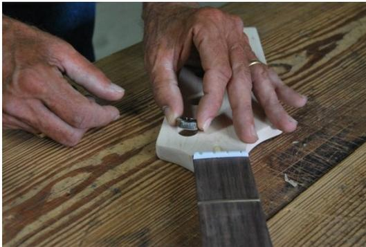
Next slide the tuning machine into the hole from the back of the headstock. **Be sure to mark and drill pilot holes for the tuning machine screws.** The Maple neck is very hard and the tuning machine screws are small and easy to strip/break. Secure each tuning machine with to the back of the headstock with the screws provided.
